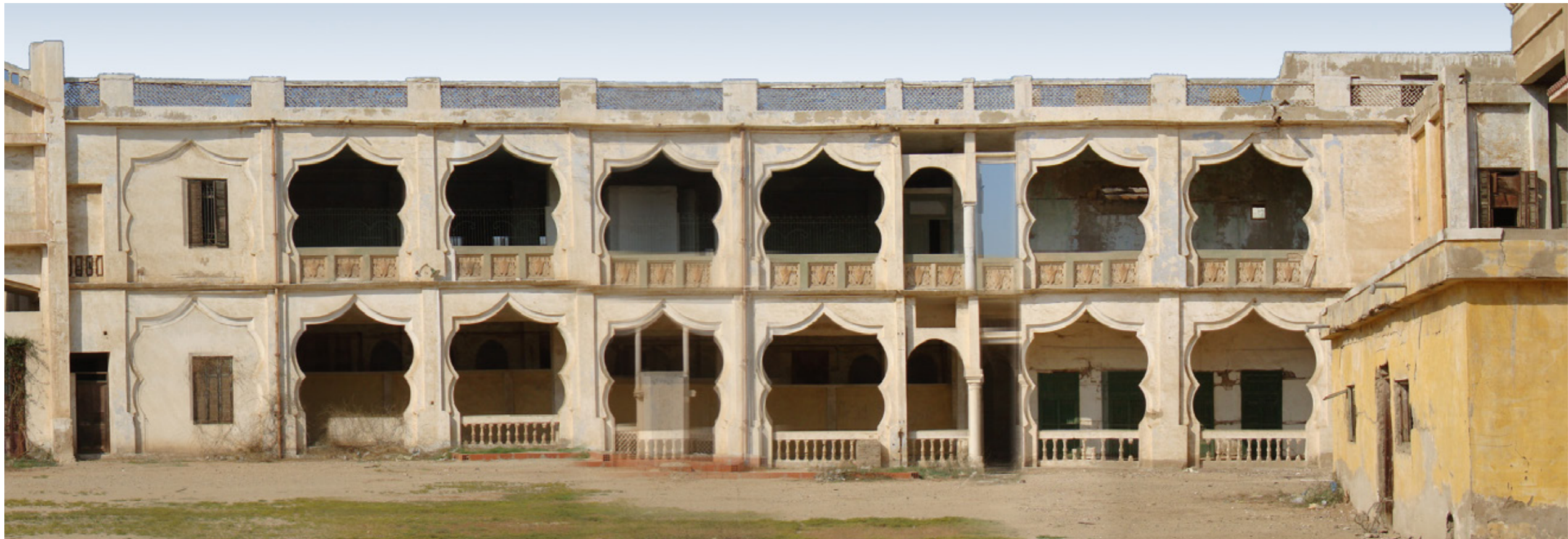
Attached pictures show the architectural study of the facades of the western building. The main feature of this façade is engraving, arches, doors and semi-circular windows
