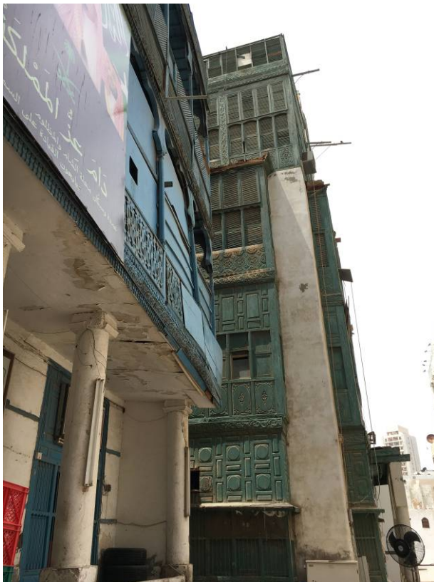
Side (left) & Back elevation (partial)
