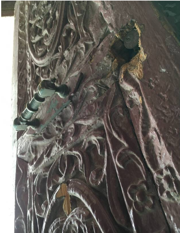
Refined sculptured wooden door, at the entrance: need for cleaning and repair, with the replacement of a few damaged elements...
