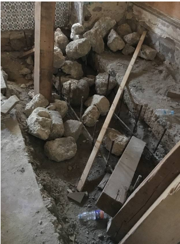
Foundation consolidation (steel-frame concrete)
